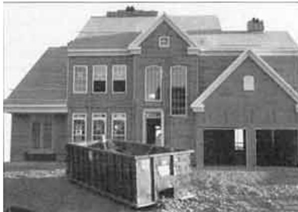
**Figure 2. The builder keeps this jobsite clean by using an onsite trash collection bin**
