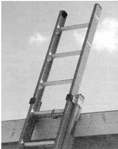
**Figure 5. When ladders are used for access to an upper level they must extend at least 3 feet above the roof surface.**
