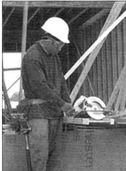
**Figure 1. This worker is preparing to cut lumber while wearing the proper personal protective equipment. He is wearing a hard hat and safety glasses, and the saw is guarded correctly. His employer has determined that he should use hearing protection.**
