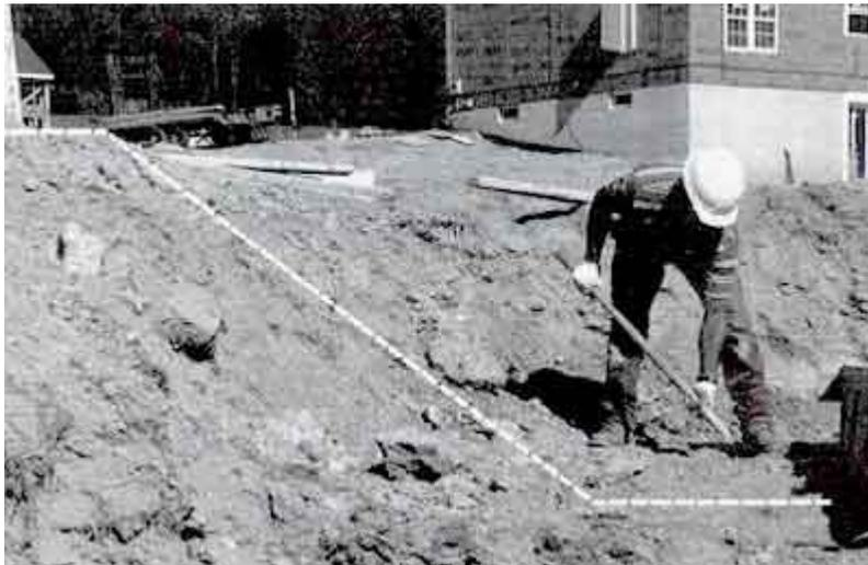
**Figure 17. The dotted line shows the profile of this excavation, as it was sloped at 1½ :1. Usually residential excavations are type C soil and will require such a slope. The spoils pile is at least 2 feet back from the edge of the excavation.**
