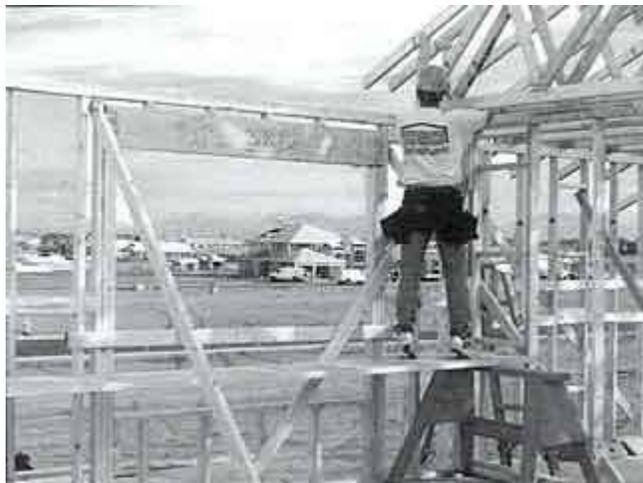
Figure 14. This worker uses a recognized safe work practice by standing on a work platform to secure the end of the roof truss.
