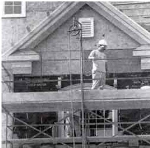
**Figure 9. Workers stand on a fabricated frame scaffold. They have ladder access to the top of the scaffold (out of view); guardrails, cross bracing, and complete planking to prevent falls. The workers are also wearing hard hats and using eye protection.**
