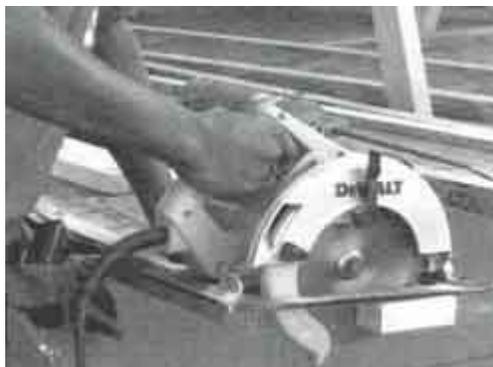
**Figure 20. This worker is using a power saw that has all moving parts, including the saw blade, properly guarded.**
