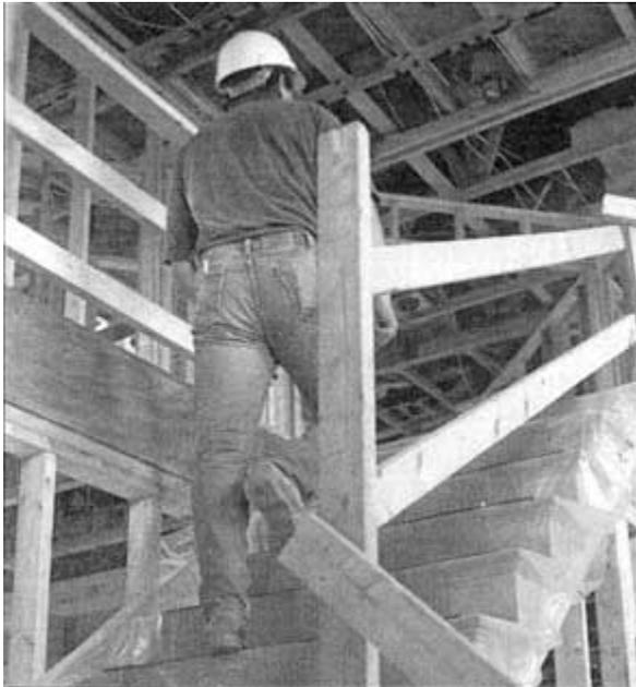
**Figure 3. Worker is walking up properly guarded steps.**
