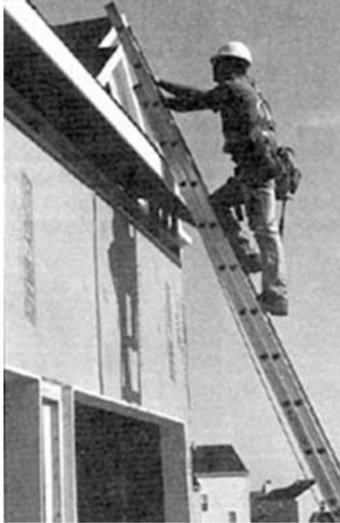
**Figure 6.** This worker is climbing a ladder set at the proper angle (4:1) with a three-point contact grip (two hands and one foot).
